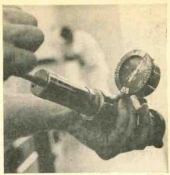
Measuring radiator cap pressure. Wrong reading could mean engine overheating.
