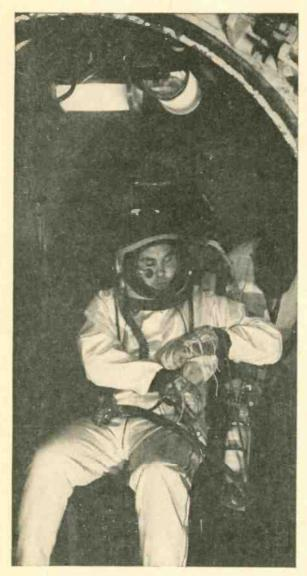
Inside chamber (above), pilot plugs leads into special suit, linking devices that monitor body functions with indicators on external panel. Pilot will be subjected to mock SST "trip," and while enroute will describe sensations to attending physicians.
